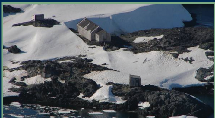
The main hut seen from the air with the emergency store in the foreground and a kennel to the rear
